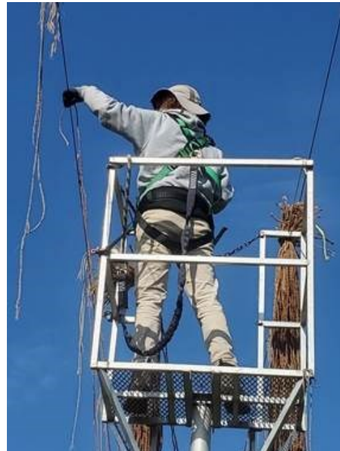
Conner Polsin using the new safety harness at Madison County hops farm, The Bineyard.
