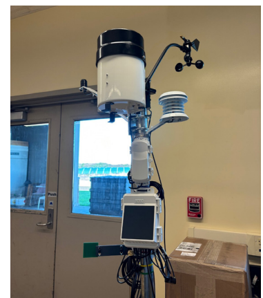
Figure 2 new Onset station ready to be installed
